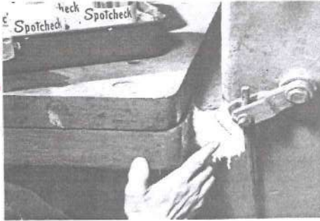
Figure 2. Spotcheck is used to locate fatigue crack in punch press frame.
